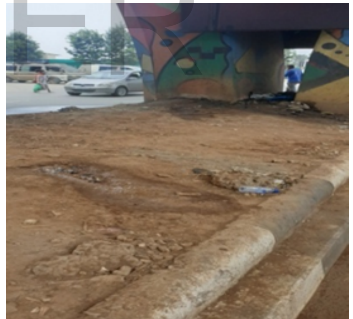
Figure 7: Picture: Under bridge uls
